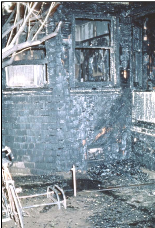
Photograph the exterior of the building to show the extent of fire damage and locations of doors and windows.
