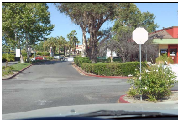
Photograph view obstructions and defective traffic control devices. This photograph was taken from inside the driver's vehicle to show a defective stop sign.
