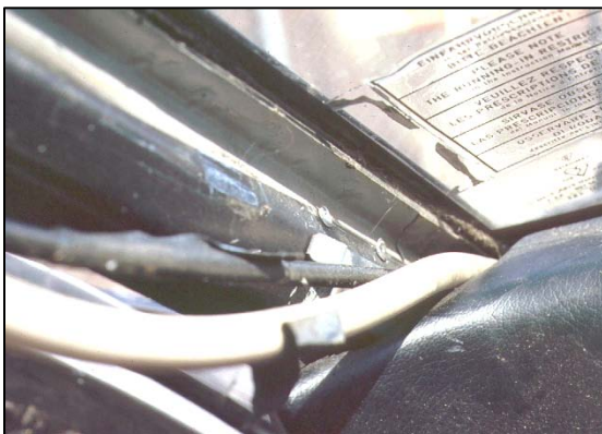
This photograph was taken to show where a vehicle identification plate had been removed. The rivets that held the VIN plate remain.
