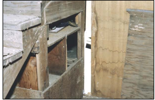
Point of entry into warehouse, exterior view.
