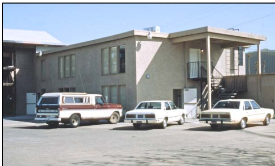
A series of photographs of this commercial burglary includes a view of the front of the office building.
