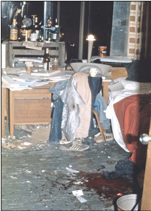
Interior view of room where the explosion occurred.
