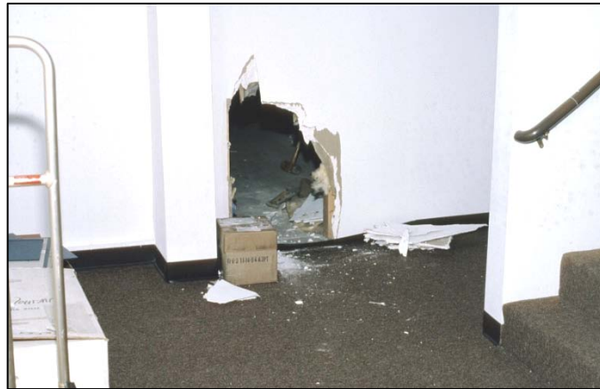
TOP LEFT: Point of entry into the office building.
