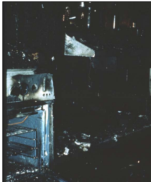
RIGHT: Fire scene photographs are often underexposed since charred walls tend to absorb, instead of reflect, light.
