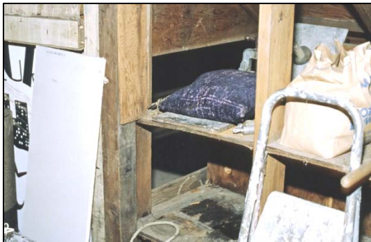
Point of entry into warehouse, interior view.
